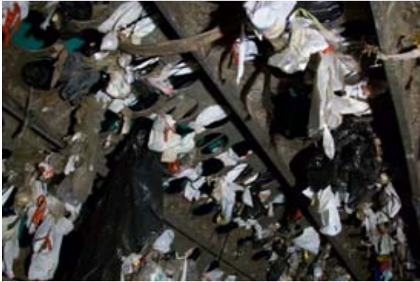
Figure 1: Sunnyvale SMART Station Trommel, clogged with plastic bags
